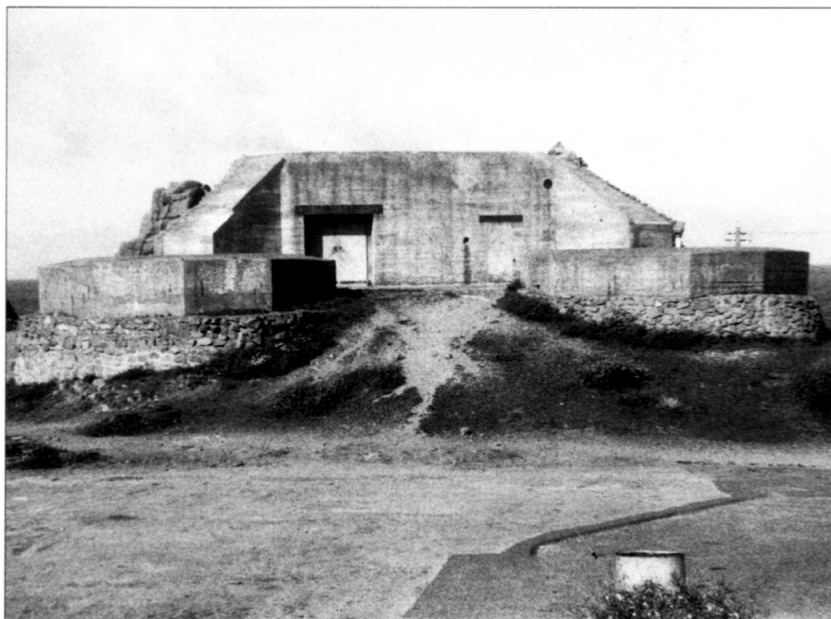
Type 606 searchlight bunker at StP Corbiere. The lights were wheeled out to the operating platforms on each side of the structure for use. (Courtesy of Michael Ginns)
