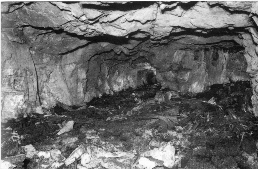
Ho 5 branch junction at southern end of tunnel. Note the remains of the wooden lining littering the floor and the exposed rock thus left. (Courtesy of Nick Catford)
