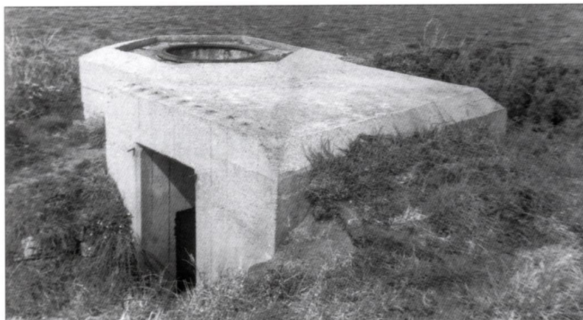
A tobruk position forming a part of the perimeter defence of Batterie Moltke, Jersey. Designated a Ringstand , it was constructed to mount a tank turret removed from a French Renault FT-17. (Courtesy of Michael Ginns)
