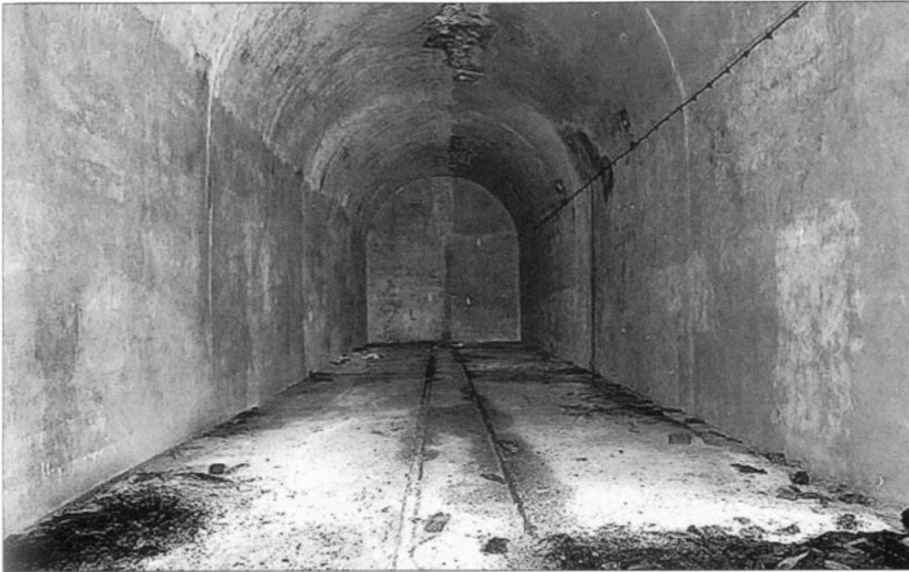
Photograph of the eastern chamber of Ho 5 Alderney, which is about 4.5m high and some 17m long. The remains of the narrow-gauge (60cm) tramway can clearly be seen and the concrete lining is in good condition. (Courtesy of Nick Catford)
